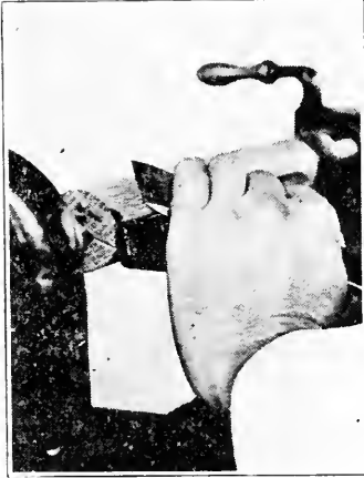
FIG. 296. USING LARGE SKEW—SECOND POSITION.
